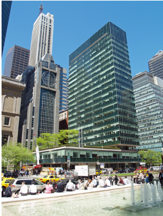
Abb. 2 | Lever House, Gordon Bunshaft, New York City, 390 Park Avenue, erbaut 1951–52
